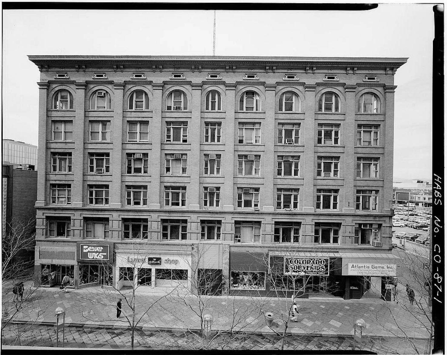
The building itself, decades later. Library of Congress
